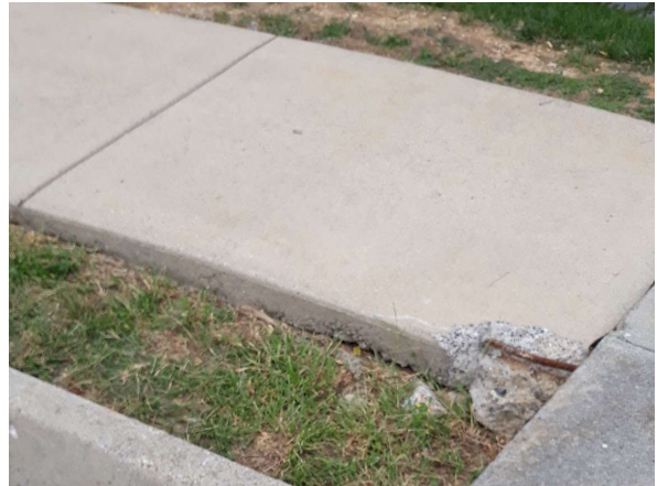
Minor damage to sidewalk
