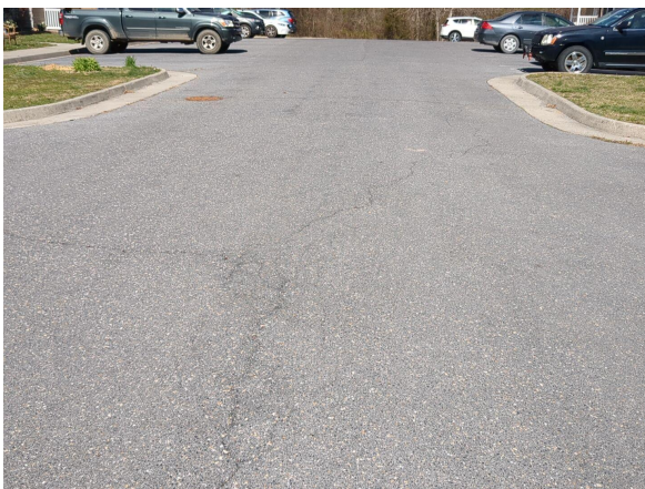
Asphalt parking - cracking and wear
