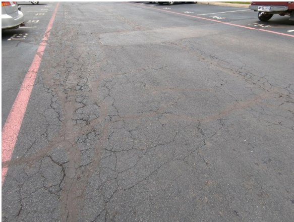
Damaged asphalt parking
