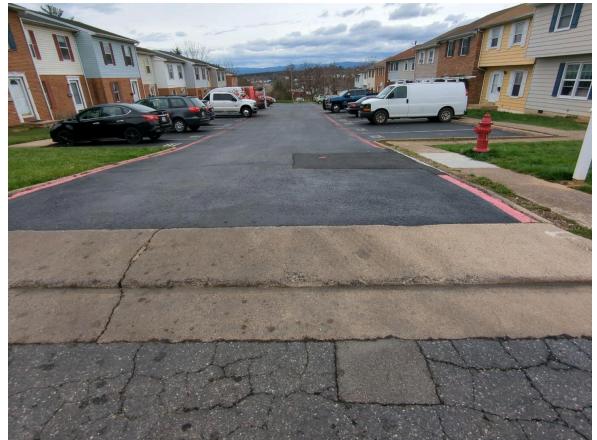
Damaged concrete apron
