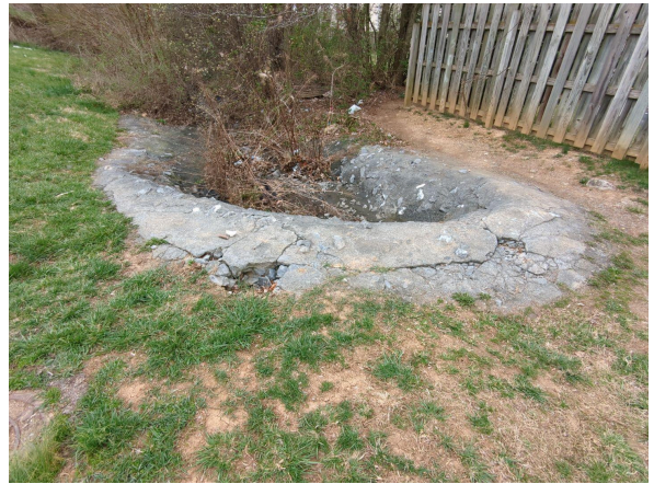
Damaged concrete at drain for stormwater area
