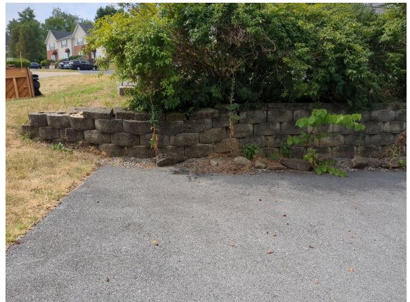
Damaged retaining wall
