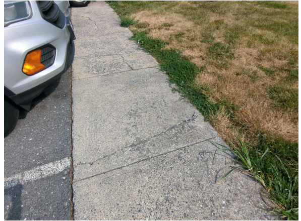
Example of damaged concrete walks
