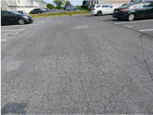
Worn asphalt parking
