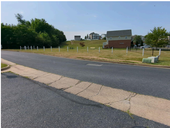
Damaged concrete apron
