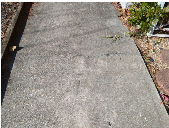
Localized crack in walk
