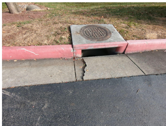
Damaged concrete curb guttering
