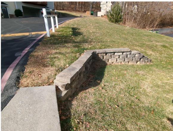
Example of retaining wall
